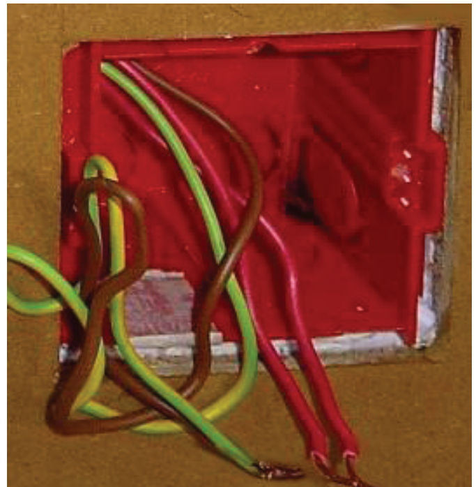
Typical wall socket box with two sets of wires: one for the main current and the other for ventilation control.
